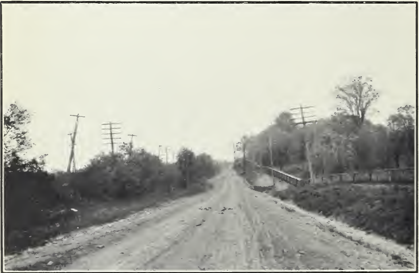
FIG. 2.—EARTH ROAD IN ALEXANDRIA COUNTY, VA., SHOWING RESULTS OF DRAGGING.
